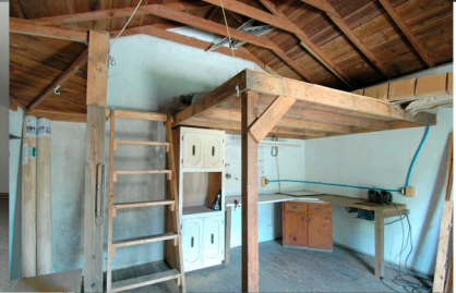
Historical Bellsouth Communications Building
